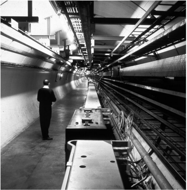
Figure 11.3. A view of the LEP tunnel. The beam travels in a pipe inside the multiple magnets that run down the centre of the picture. To the left is the track for a monorail that runs the length of the tunnel. To the right are various servicing and cooling ducts. (Courtesy CERN.)
